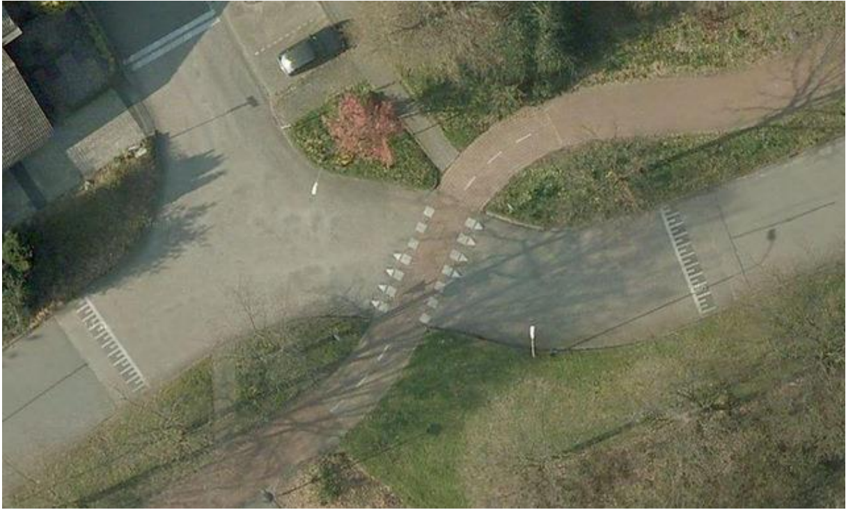
Figure 20 Cycle priority crossing of a minor road (Source: David Hembrow)
