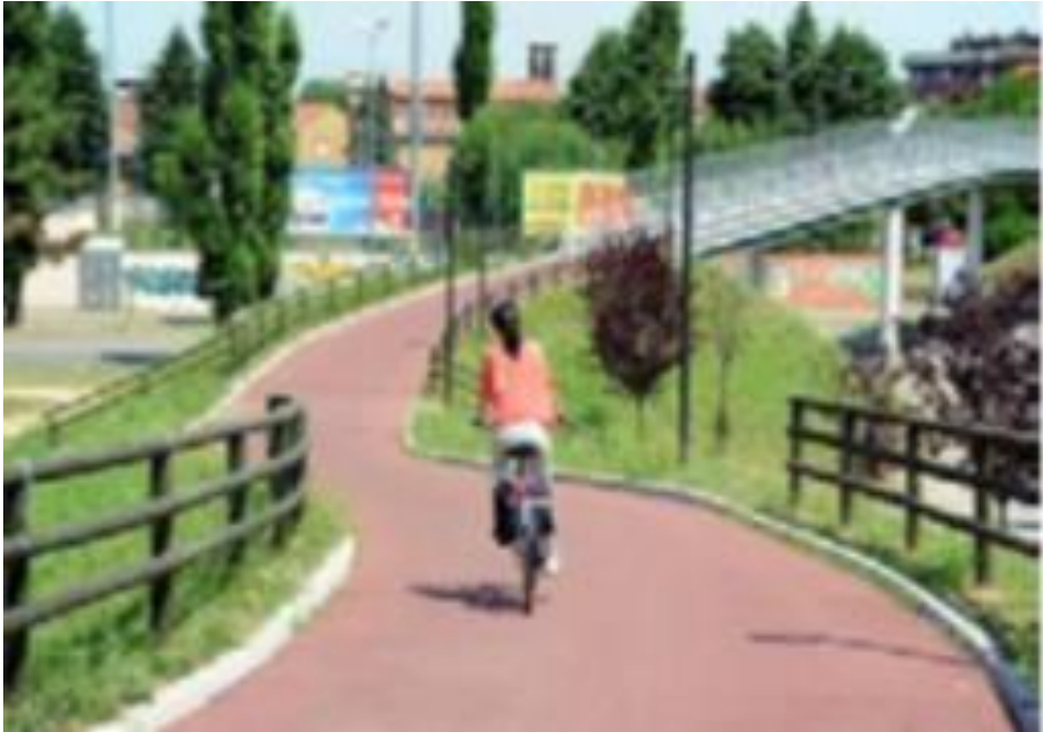
Figure 12 A bicycle bridge in Milan
