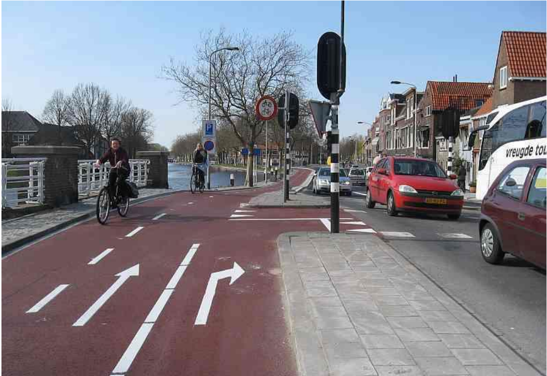
Figure 16 Two way-two lane bicycle path with right turn lane in Amsterdam (Source: Pascal van den Noort)
