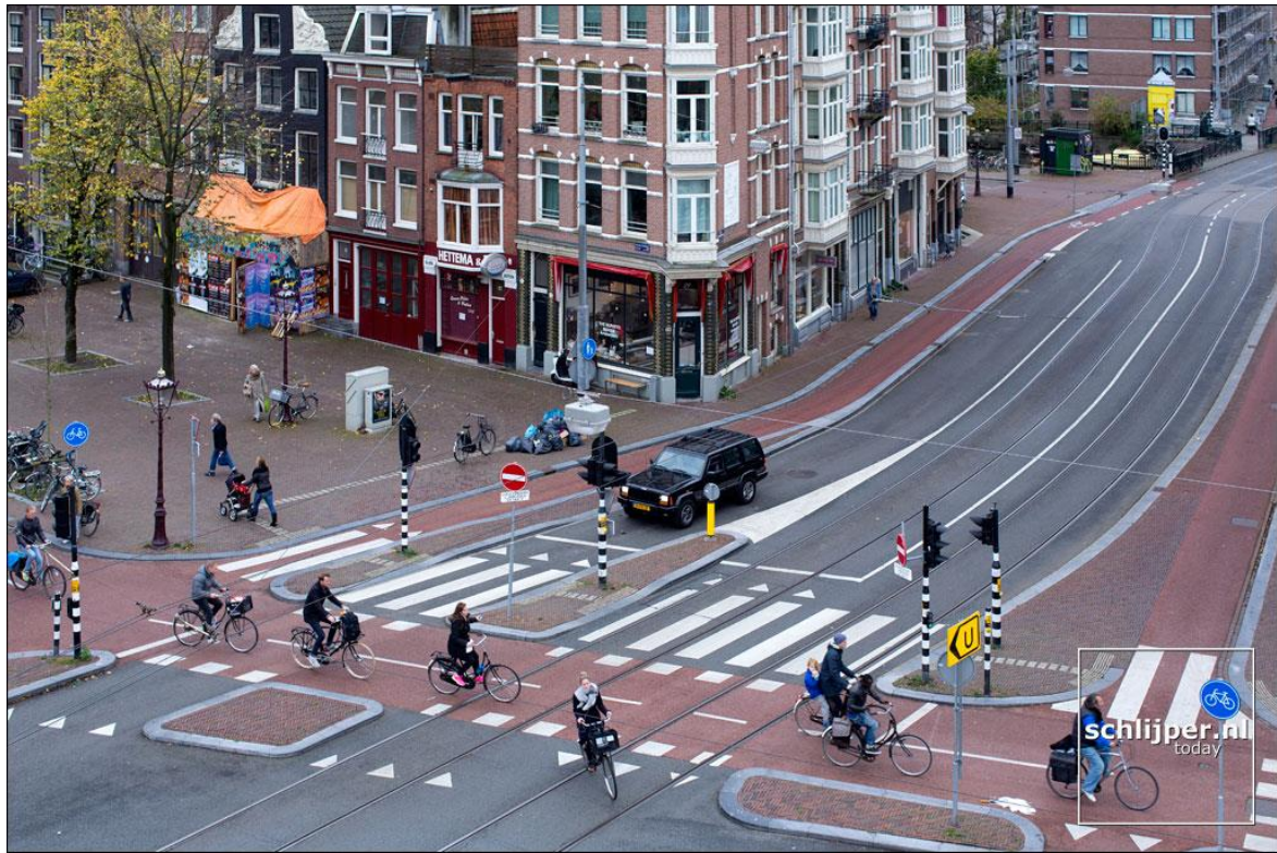
Figure 18 A protected intersection in Amsterdam (Source: Thomas Schlijper)
